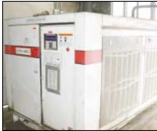
GARDNER DENVER MODEL ST-150 150 HP ELECTRA SAVER II ROTARY SCREW AIR COMPRESSOR
