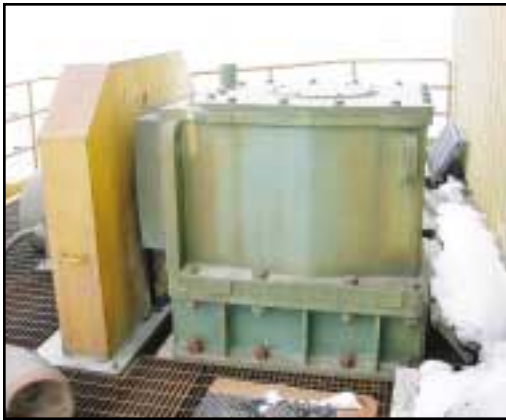
LIGHTNIN MODEL 783-Q-150 RIGHT ANGLE TANK AGITATOR
