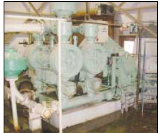
GEHO MODEL ZPM-700 200 HP DC PISTON DIAPHRAGM PUMP
