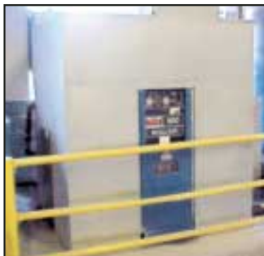
WORTHINGTON ROLLAIR MODEL 100 100-HP ROTARY SCREW AIR COMPRESSOR
