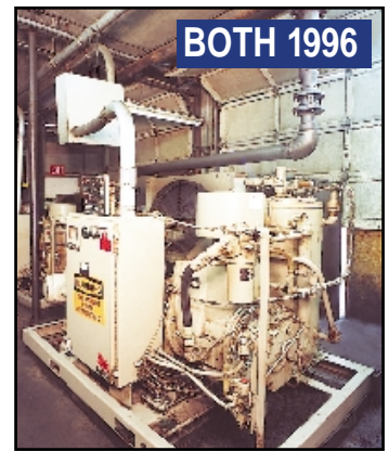
LEROI WE200SSIIA 200-HP ROTARY SCREW AIR COMPRESSORS
